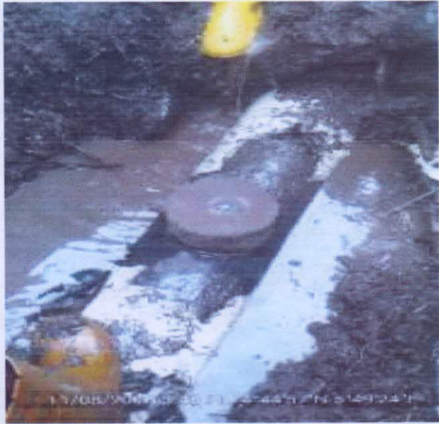
FIG B: Incident point after repairs (Coning)
